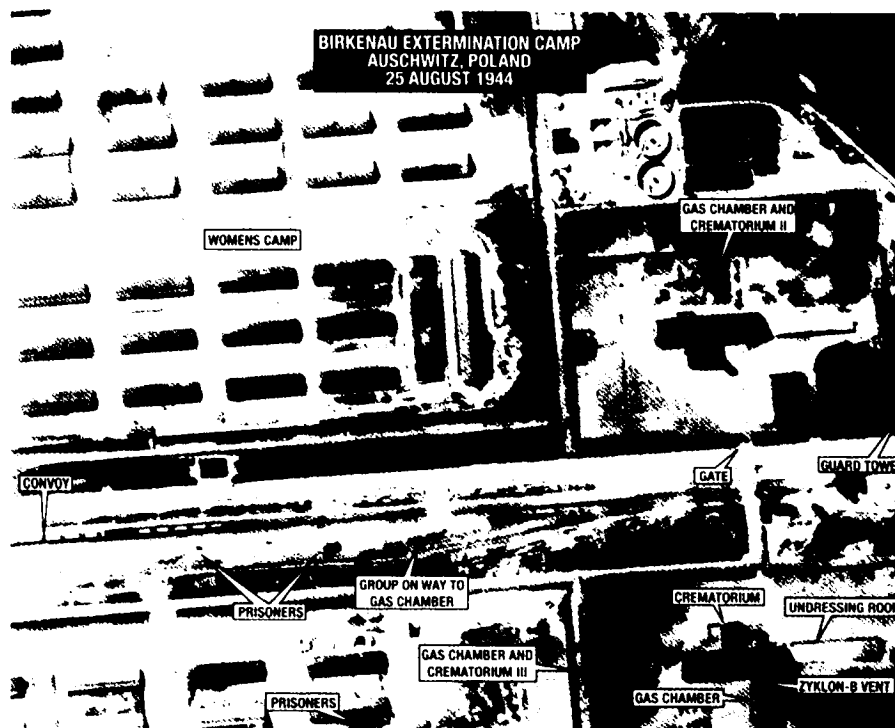
This aerial photograph allows us to identify some of the features of the Auschwitz death camp.
